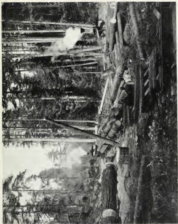
FIG. 80. LOADING LOGS WITH GINPOLE. [By courtesy of British Columbia Government.]
